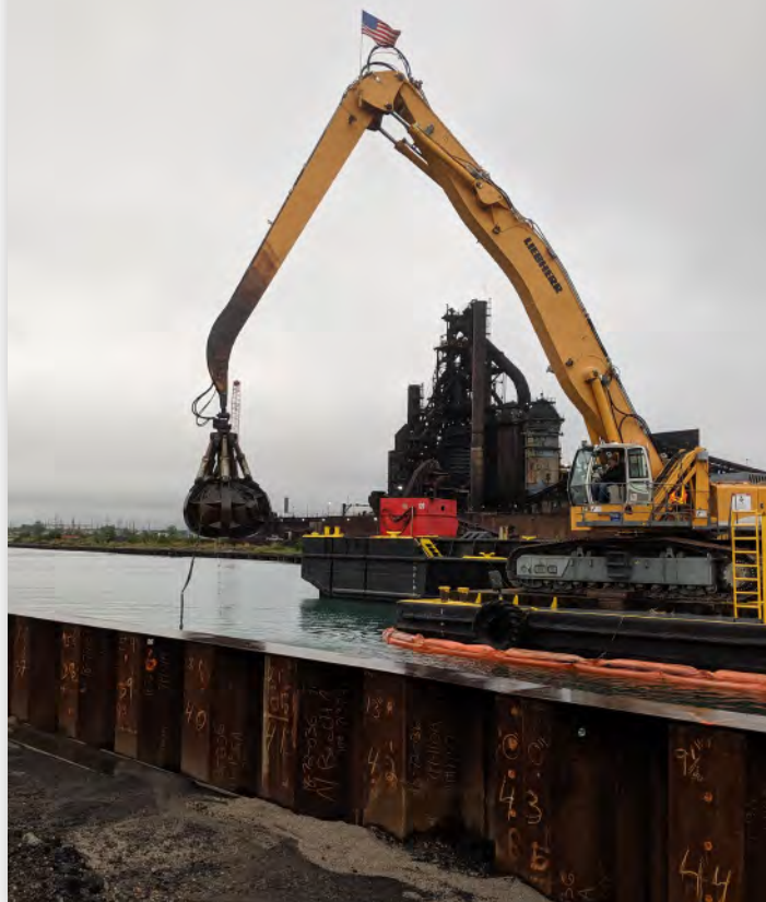
Dredging of contaminated sediment is part of remediation efforts in the Rouge River Area of Concern. Photo courtesy of EGLE.
